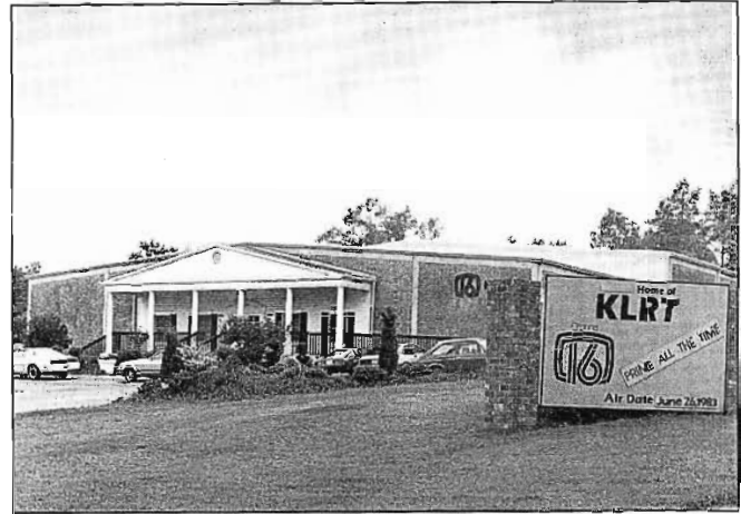
Studio and administration building
